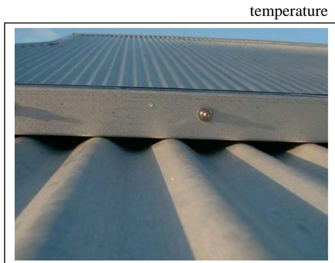
Figure 5 Air gap below panels on my system
